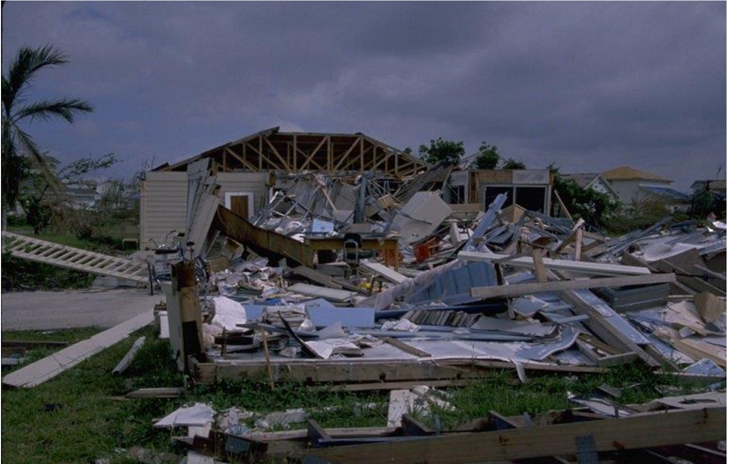
Damage from Hurricane Andrew in Miami-Dade County, Fla., in August 1992. (FEMA News Photo)
